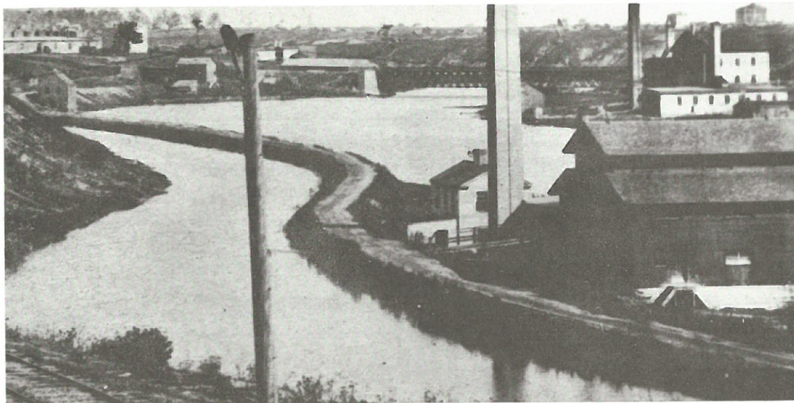
The Milwaukee and Rock River Canal as it looked about 1850 shortly before it was filled in. The building with the tall smoke stack in the right foreground was the old Ludington and Garland Paper Mill, one of many industries that utilized the canal as a source of water power. (Courtesy Milwaukee County Historical Society)
